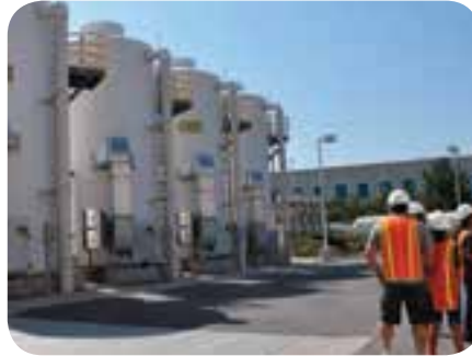
See how your water is treated and delivered by attending a quarterly facility tour.
